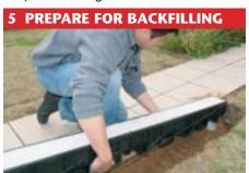
Mask along the grates over entire run length. Lower channel assembly, seal to drain pipe and pack to correct level.
