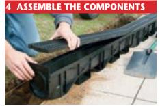
Connect channels together and fit end caps.
