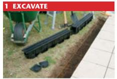
Excavate trench and fix a line to determine the alignment and finished height of proposed
