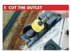
Cut out preformed outlet located in base of the channel to allow connection to drain pipe.
