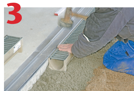
Lay channels starting at outlet. Set a string line at required height to ensure level. Seal joints if required.
