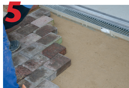
Install pavers or finish pavement surround to required level. Should be 1/8" above grate.
