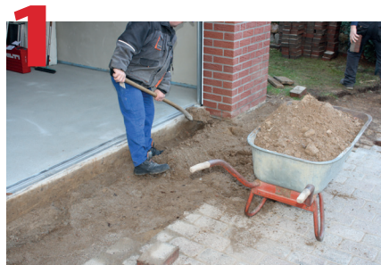
Excavate area to allow room for channels/catch basin and 4" of concrete on all 3 sides.
