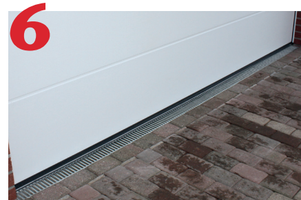
Clean away debris, remove protective plastic.
