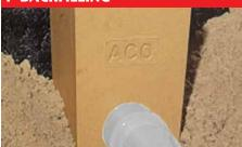
Connect drainage pipe, check for leaks before backfilling.
