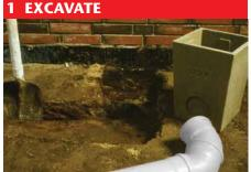
Dig hole to fit PointDrain and necessary pipe-work.
