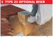
Add riser (if required) and connect inlet pipe (if required). Surround PointDrain with concrete.
