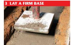
Lay 100mm thick concrete bed, ensure unit is level.
