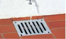
Ensure finished surface is 3mm higher than the grate to assist water drainage.
