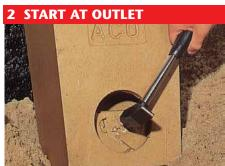
Drill out/cutout holes for pipe connection.
